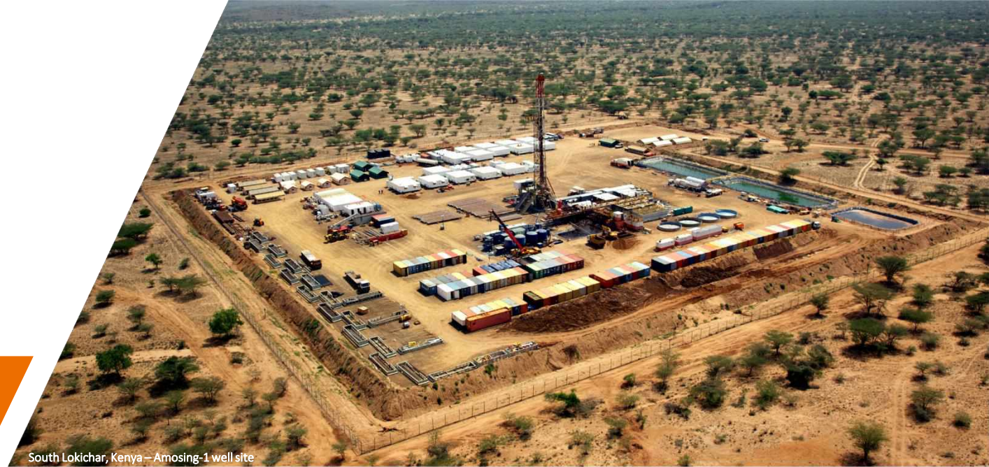
South Lokichar, Kenya – Amosing-1 well site
